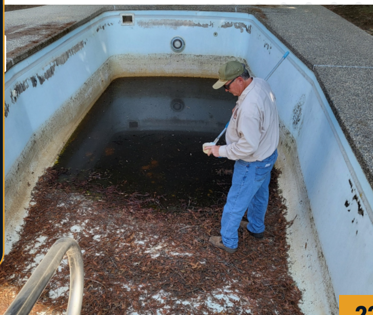
Field technician Eric Ferguson inspecting an unmaintained swimming pool.
