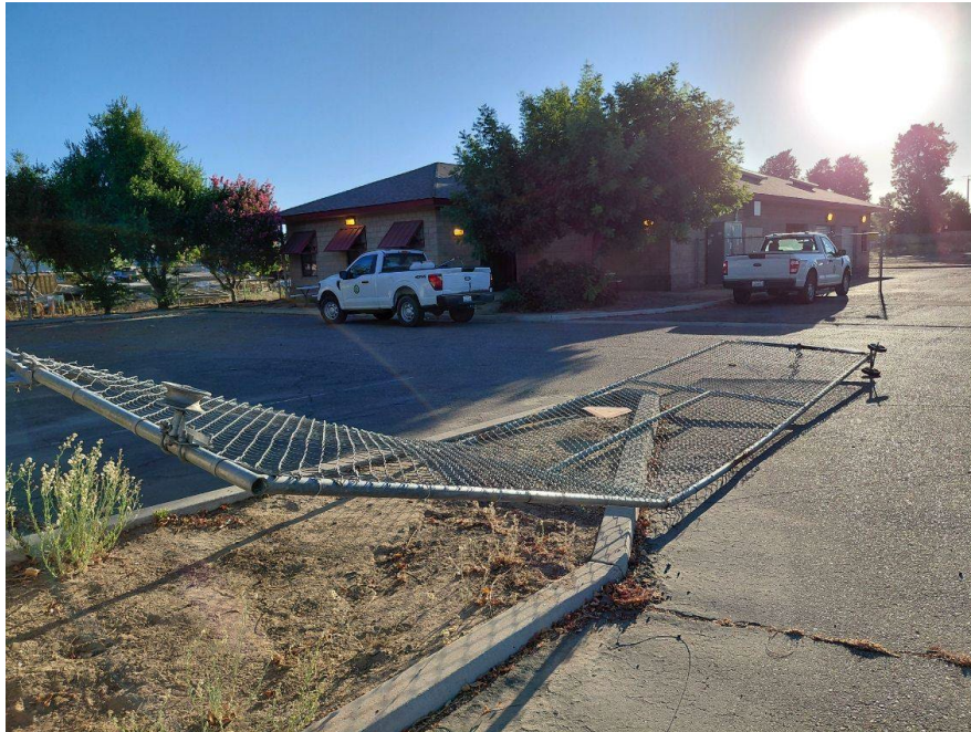
Collapsed chain-link swing gate at Clovis facility entrance.
